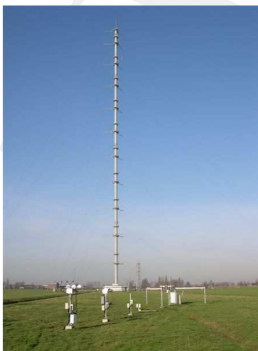
FIGURE 1: The 213m tower at the Cabauw site in The Netherlands, with the Baseline Surface Radiation Network (BSRN) station in the foreground.
